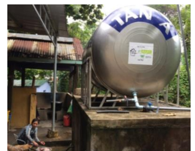
Water tank and "happy tap" for hand-washing in the Nam Giang schools
